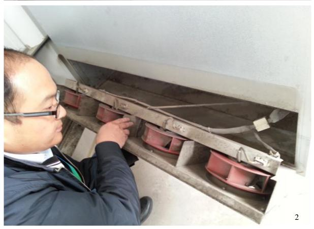
Step 6: Cut the cable ties which fixing the ambient sensor, then pull the sensor cable out of the cover.
