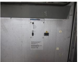
Step 2: Remove the cover of PCBA by T20 screw driver, and then unplug the connector of sensor.
